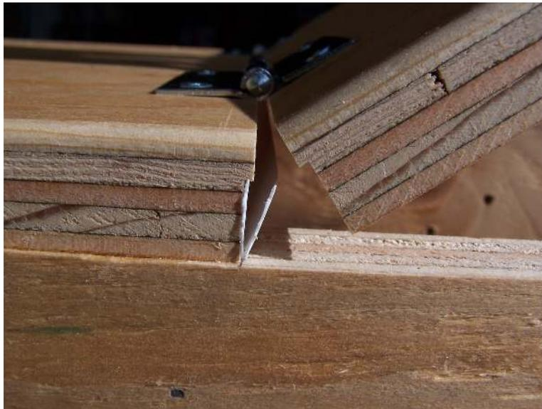
The weather stripping used is V-Flex Weather Strip which can seal gaps up to 3/8". One side of the stripping has an adhesive to hold it in place.
