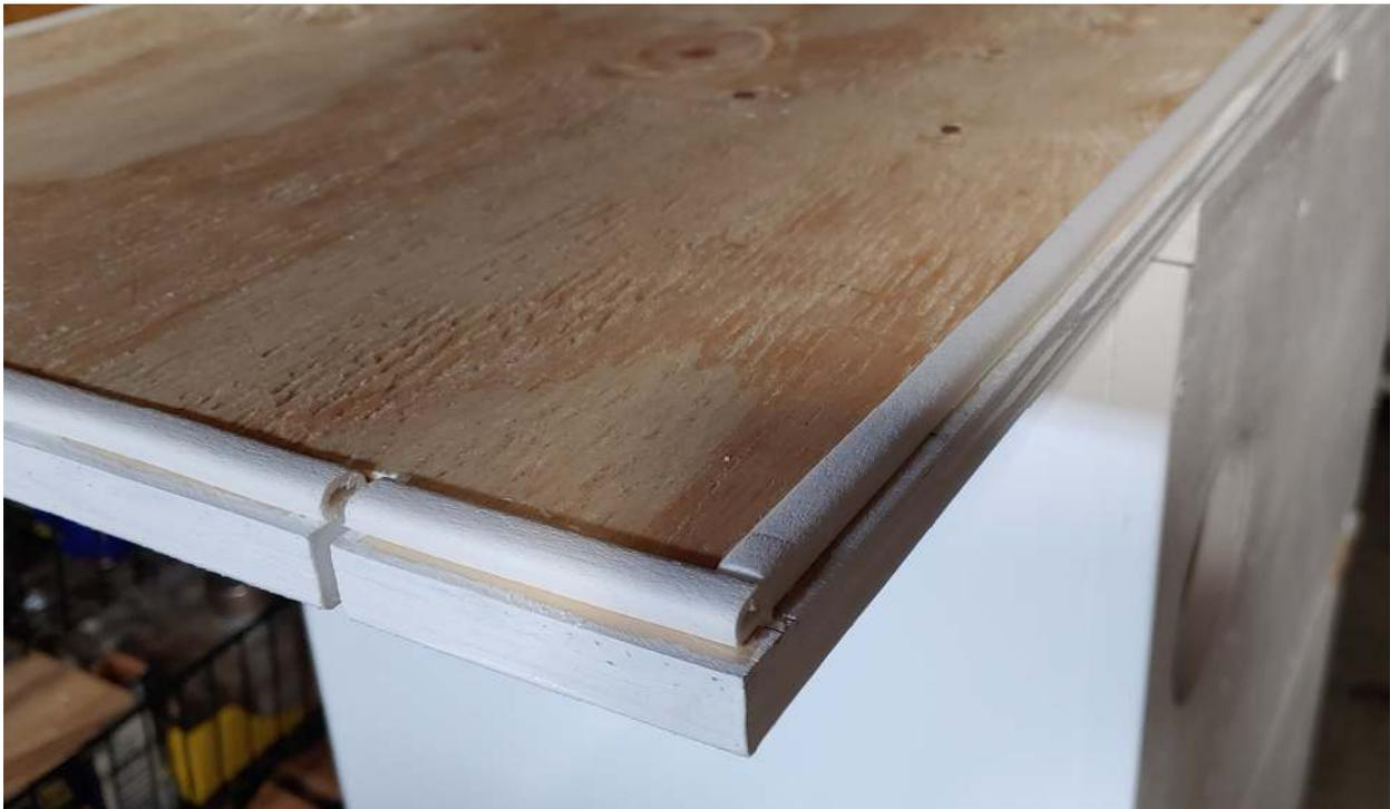
The weather stripping used is a self-adhesive rubber foam seal\*. One side of the stripping has an adhesive to hold it in place.
