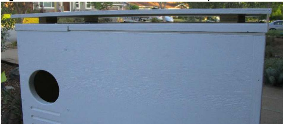
**Figure 2: Installed Sun Shield**
