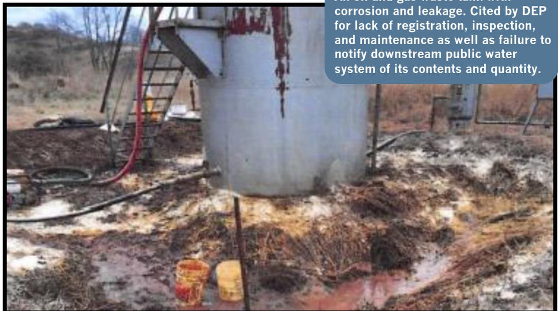
An oil and gas waste tank with corrosion and leakage. Cited by DEP for lack of registration, inspection, and maintenance as well as failure to notify downstream public water system of its contents and quantity.
