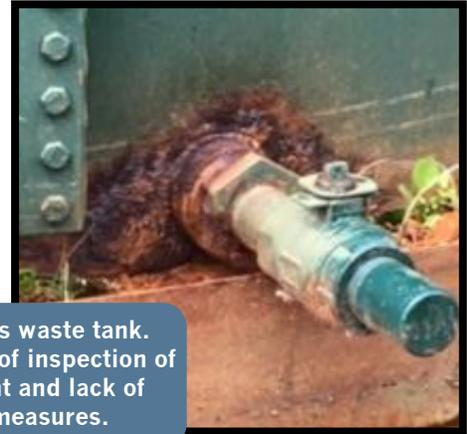
A corroding oil and gas waste tank. Cited by DEP for lack of inspection of secondary containment and lack of corrosion prevention measures.
