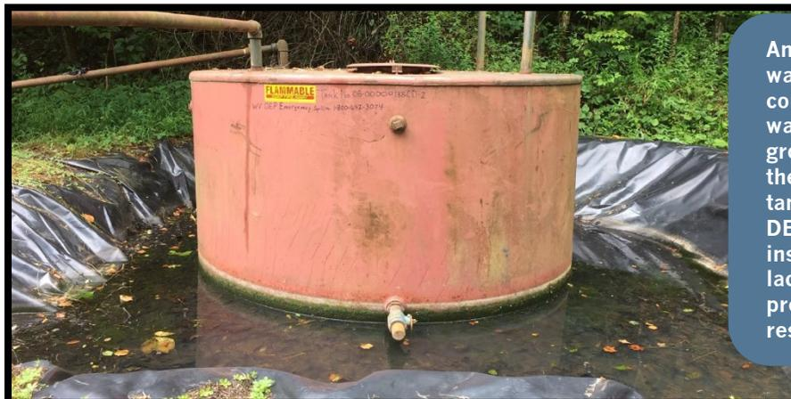
An oil and gas waste tank in contact with water, with moss growing around the bottom of the tank. Cited by DEP for lack of inspection and lack of spill prevention and response plan.
